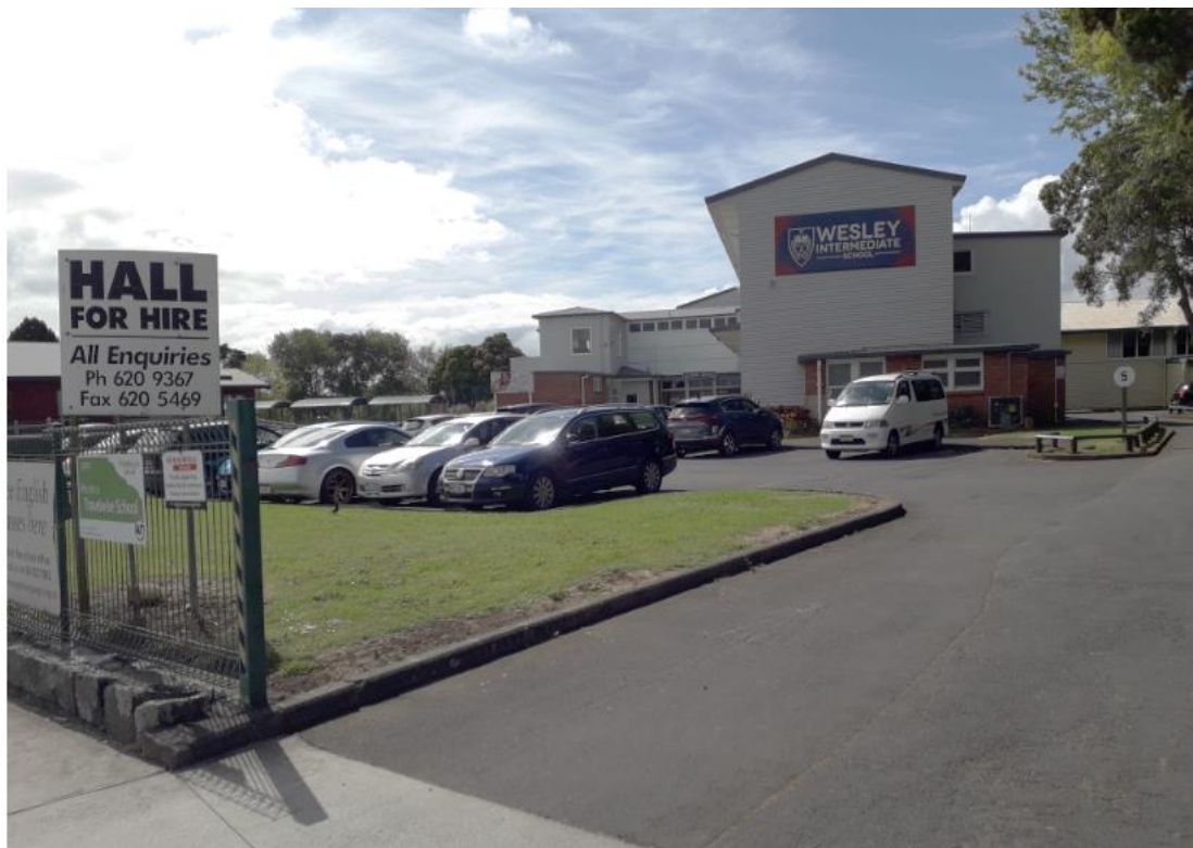
Figure 4: The main entry to the school from Sandringham Road Extension
